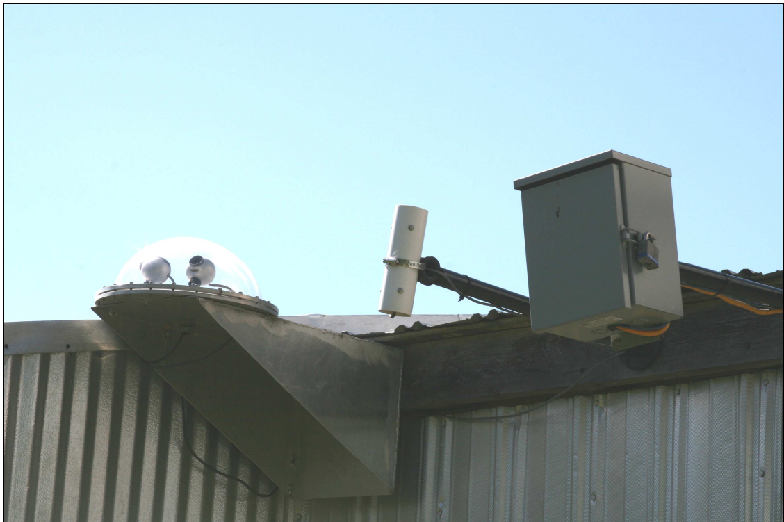
FIG. 66. From left to right, the sky webcams, Boltwood cloud sensor, and SBIG AllSky/Meteor Camera. All are mounted outside of DSO-14's control room. (Author)
