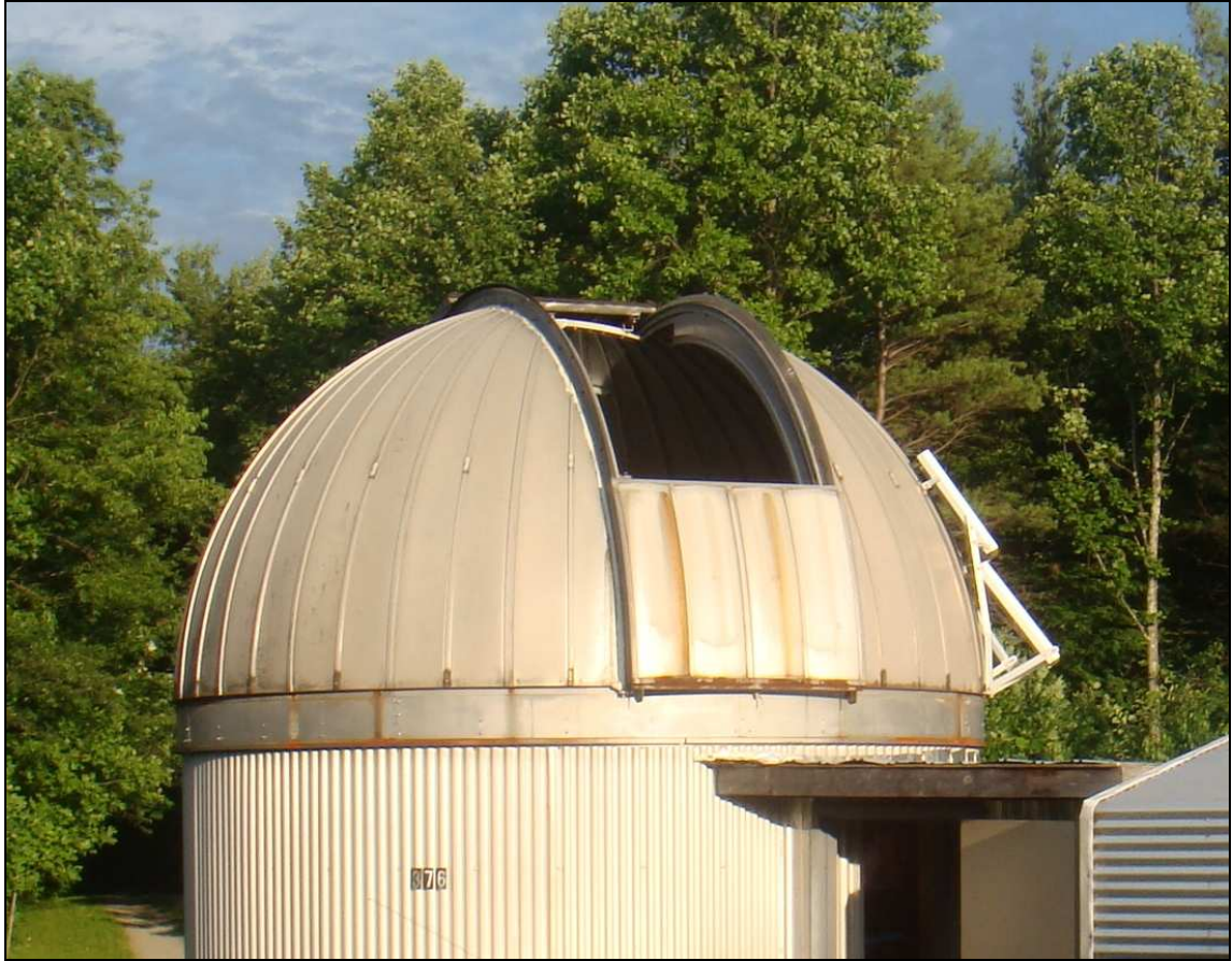
FIG. 29. DSO-14's Ash dome. The bottom of the shutter drops down by use of hand crank. However, we hope to have that motorized in the near future. (Author)
