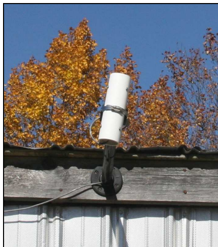
FIG. 73. The Boltwood cloud sensor uses infrared sensors to determine cloud conditions at DSO. (Author)
